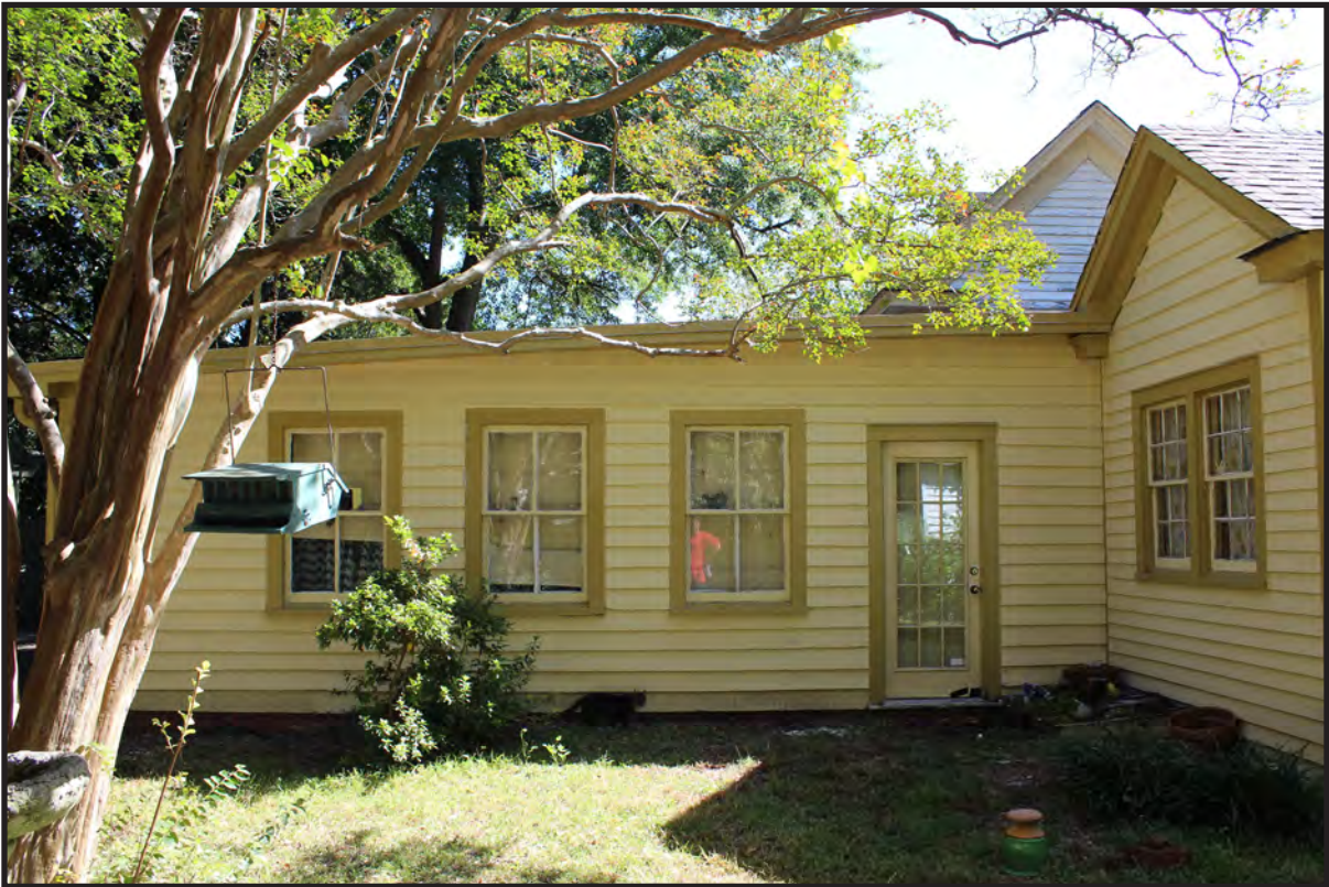
Figure 34: L. S. Hardee House, North Addition, Looking East.
