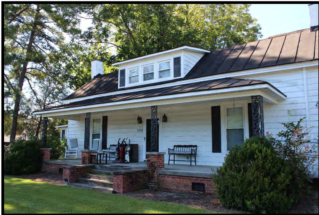
Figure 3: Edwards House, Looking South.
