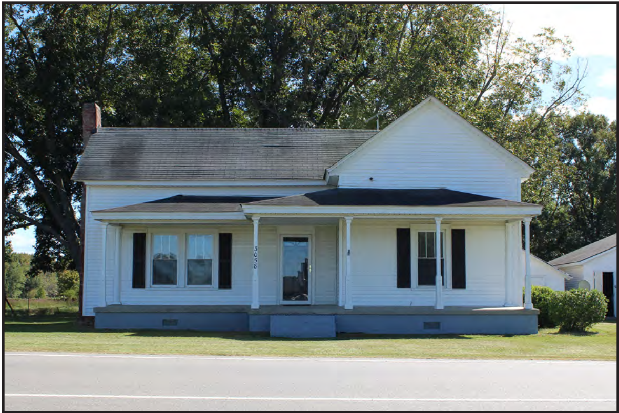
Figure 45: Ca. 1920, 3058 Portertown Road, Greenville, North Carolina.
