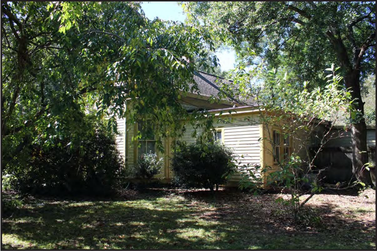
Figure 29: L. S. Hardee House, Cut-away-bay and North Additions, Looking Southwest.
