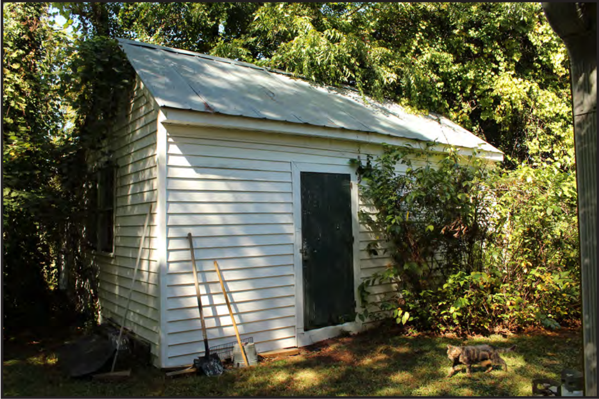
Figure 40: L. S. Hardee House, Ancillary Structure, Looking Northwest.
