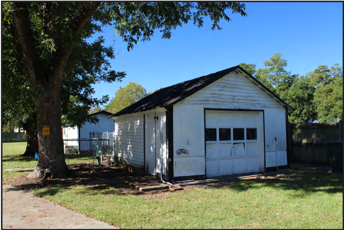
Figure 17: Edwards House, Garage, Looking West.
