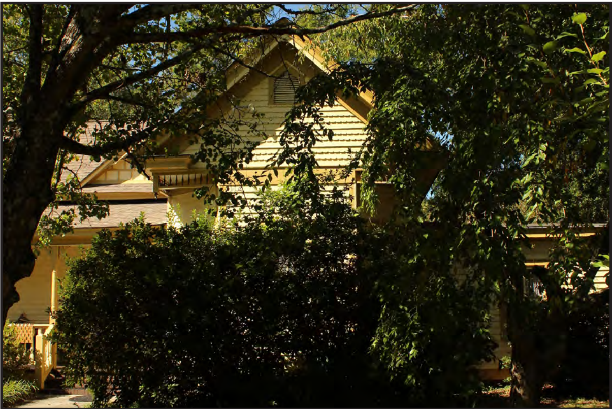
Figure 28: L. S. Hardee House, Front Gable, Looking West.
