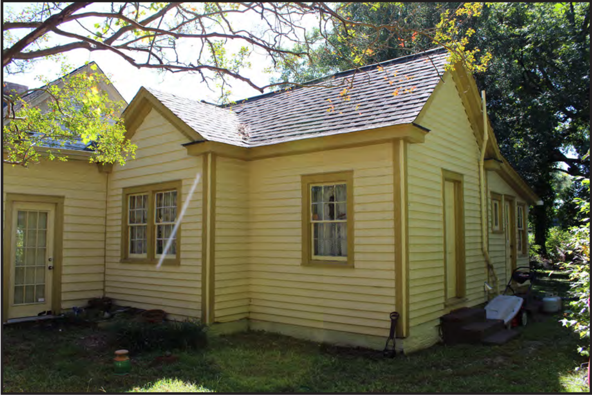
Figure 33: L. S. Hardee House, West Addition, Looking Southeast.
