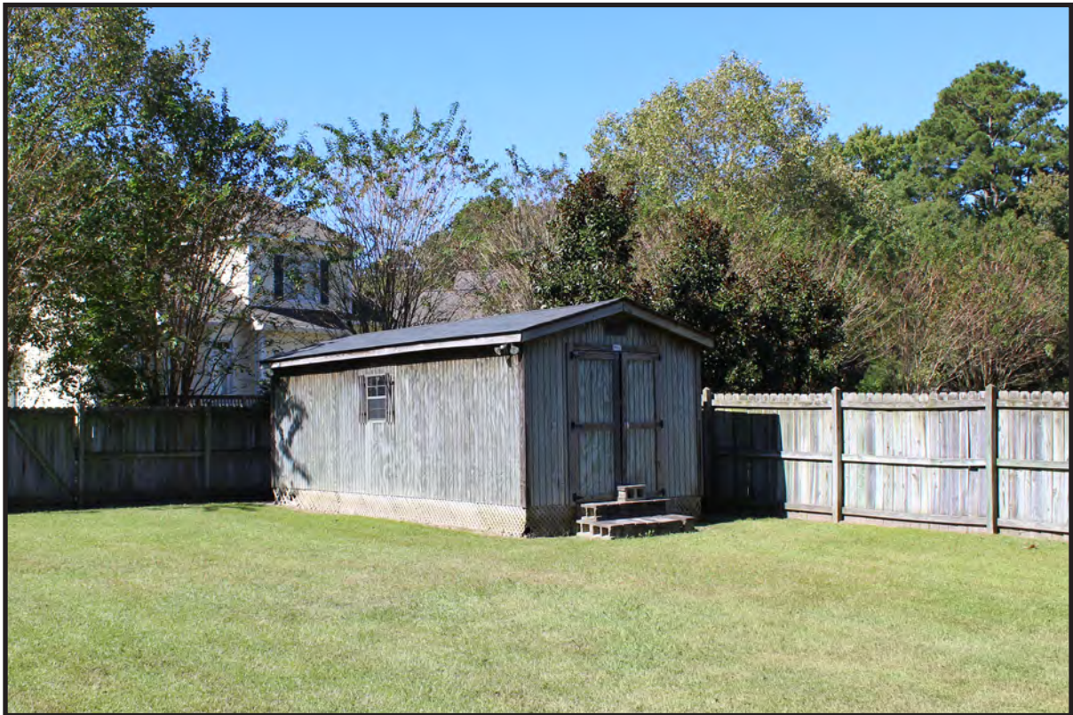
Figure 14: Edwards House, Shed, Looking West.
