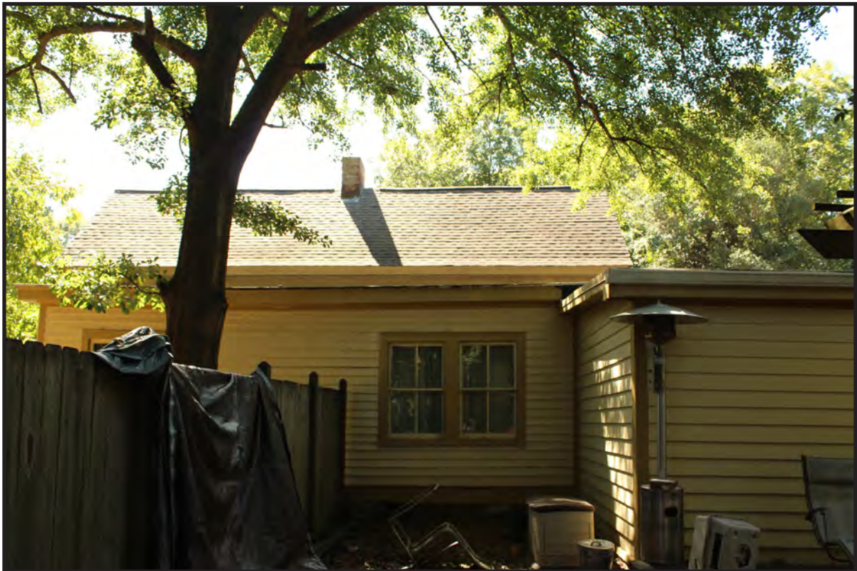
Figure 38: L. S. Hardee House, North Additions and Roof of Original Dwelling, Looking South.
