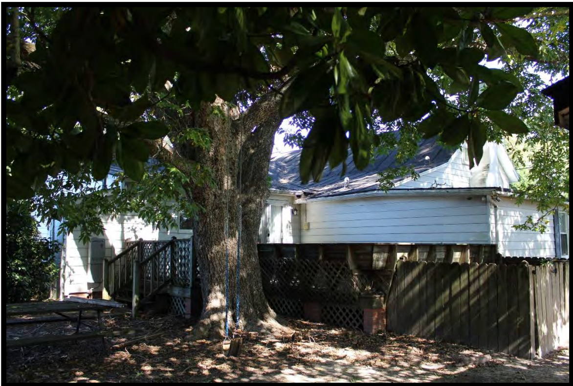
Figure 8: Edwards House, Southeast and Southwest Additions and Deck, Looking North.
