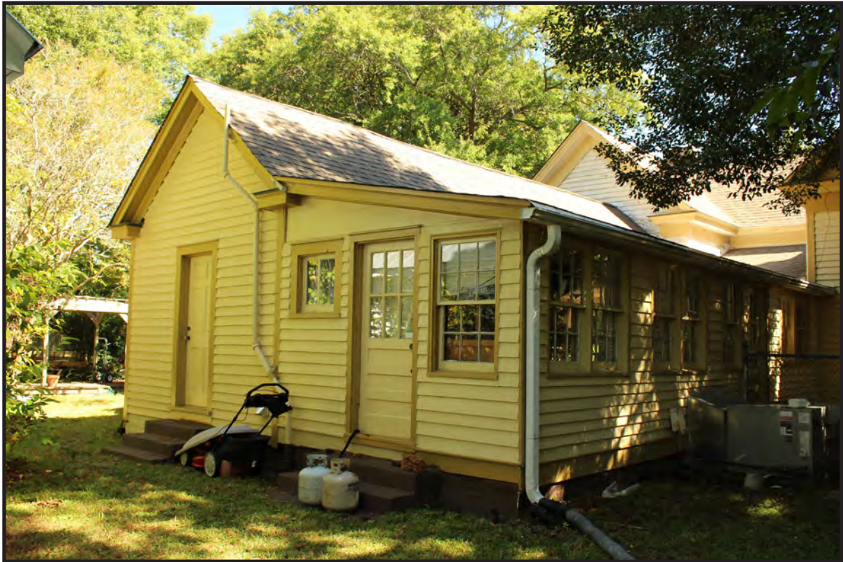
Figure 32: L. S. Hardee House, West Addition and Original Gable, Looking Northeast.
