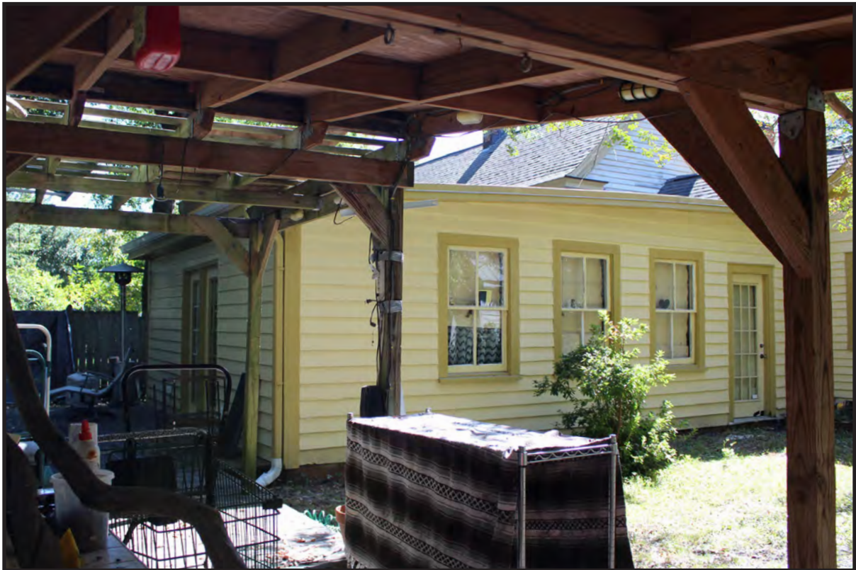
Figure 36: L. S. Hardee House, North Addition, Looking Southeast.
