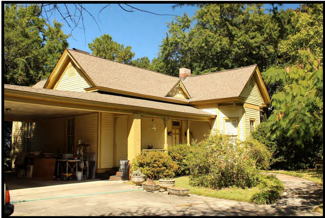
Figure 25: L. S. Hardee House, Looking East.
