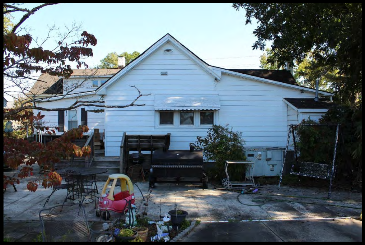
Figure 9: Edwards House, Southwest Additions, Looking Northeast.
