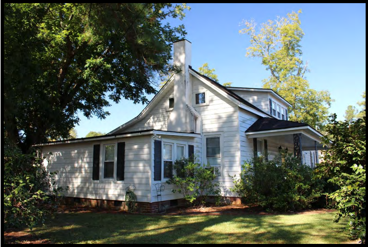
Figure 7: Edwards House, Original Exterior Chimney and Southeast Addition, Looking West.
